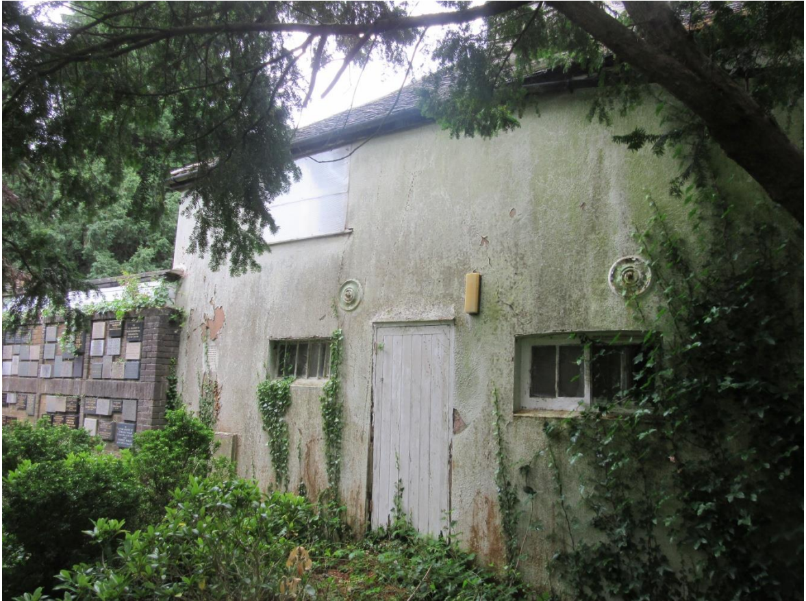
Figure 22: Rear (east) elevation of Church House.
