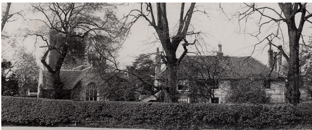
Figure 14: Church House during the early 20 th century, pre-1910 (Barnet Museum).
